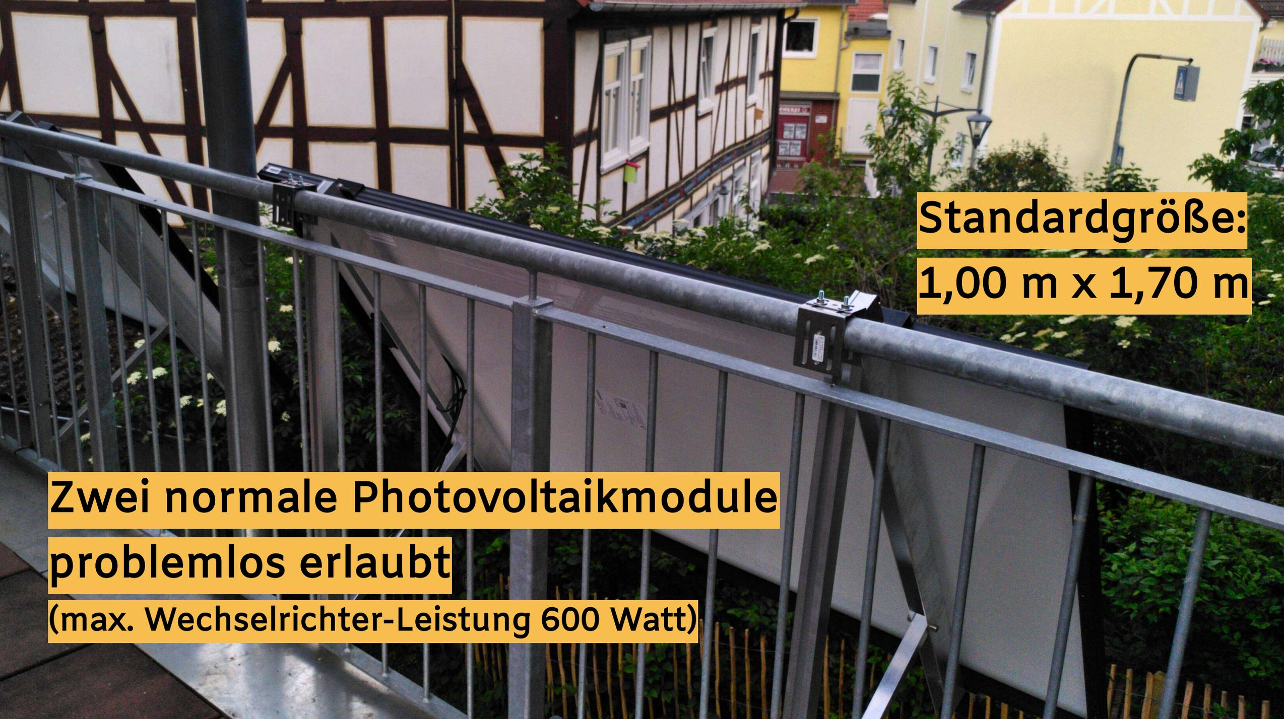
The image shows a balcony railing with two photovoltaic modules mounted on it. The railing is made of metal and has a glass panel. The modules are connected to the railing with metal brackets. In the background, there are residential buildings, including a half-timbered house and a yellow building. The scene is outdoors with some greenery.
